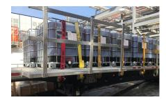
The F-500 Encapsulator Agent Concentrate Control Supply systems with 3% ratio controllers, were commissioned, tested and approved. 22,500 gallons of F-500 EA were allotted for initial start-up testing and bladder tank operation. The system is based on a 2600 gpm water flow and 30 minutes of enhanced and properly proportioned F-500 EA to protect the under turbine lube oil and transformer areas from fire.
