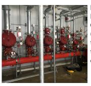
Hazard Control Technologies' F-500 Encapsulator Agent Concentrate Control Supply (CCS) Systems were chosen to protect multiple steam turbines and gas turbine compressors.
